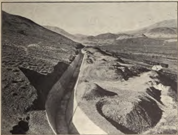
TRUCKEE IRRIGATION CANAL, NEVADA.
